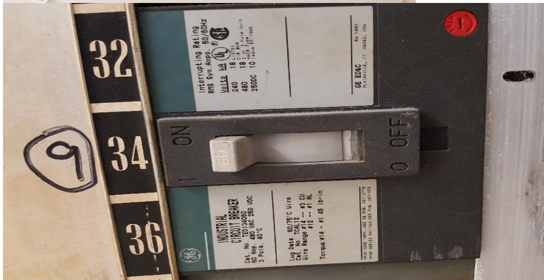
Current Typical installation of 3 pole 60 amp breaker serving the HVAC units in the residential units of the building.
