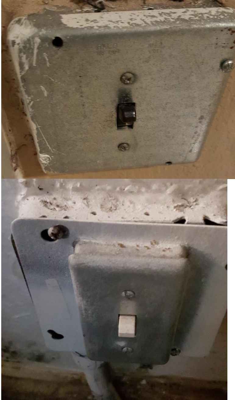
Figure 1: Existing Typical HVAC Means of Disconnect
