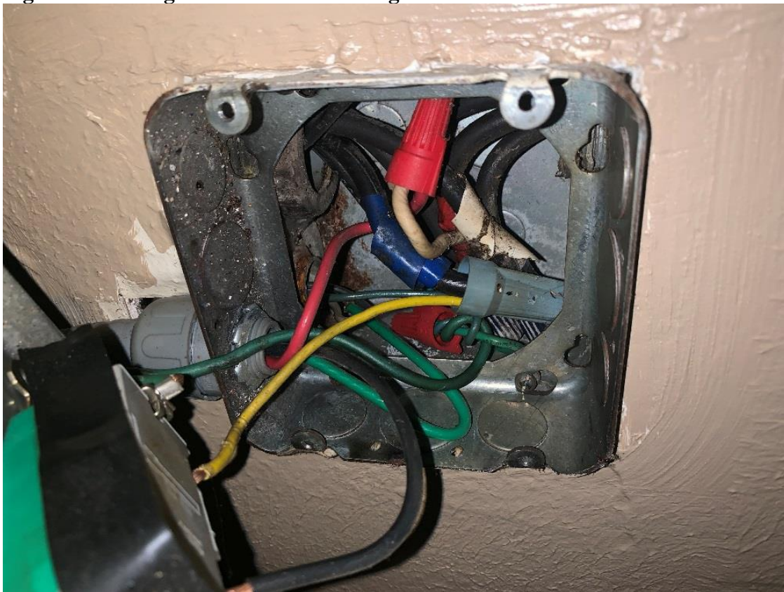
Figure 3: Existing Branch Circuit Wiring
