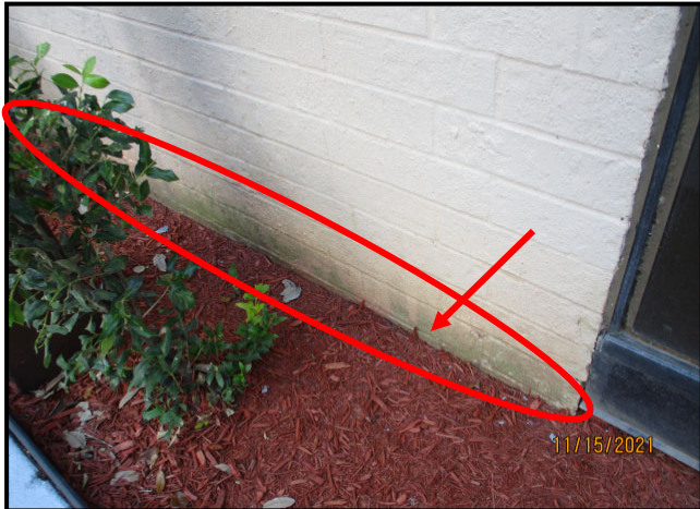
43. NO VISIBLE WEEPS AT BASE OF BRICK VENEER
