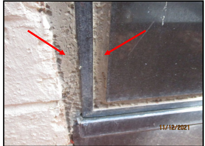
14. DETERIORATED SEALANT AT WINDOW PERIMETER, AND BETWEEN INSULATED GLASS UNIT AND FRAME
