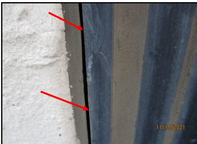
23. DISBONDED SEALANT AT WINDOW PERIMETER
