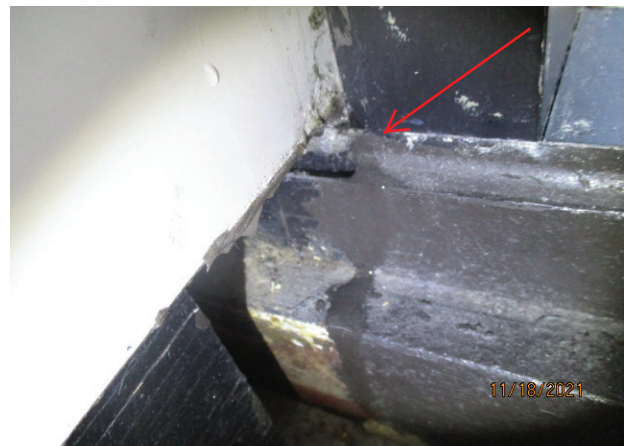
72. SPECIMEN 3.03: WATER INFILTRATION BETWEEN WINDOW FRAME AND PTAC UNIT
