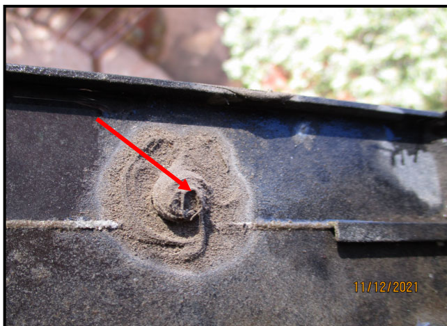
47. DETERIORATED SEALANT AROUND FASTENER IN WINDOW FRAME
