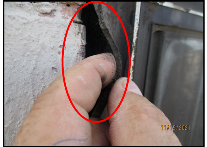
26. DISBONDED SEALANT AT WINDOW PERIMETER
