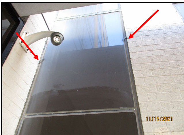
41. GLASS APPARENTLY RETAINED WITH SECTION OF PLASTIC SHIM
