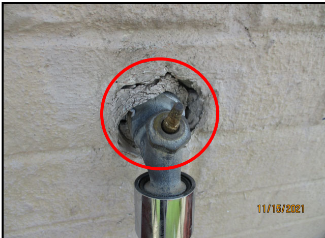
33. DETERIORATED SEALANT BETWEEN WALL PENETRATION AND BRICK UNITS
