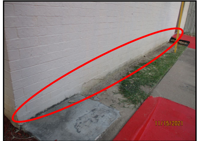
44. NO VISIBLE WEEPS AT BASE OF BRICK VENEER
