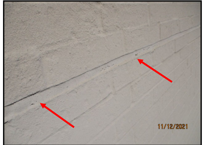
32. DETERIORATED SEALANT IN HORIZONTAL JOINT BETWEEN ADJACENT BRICK UNITS
