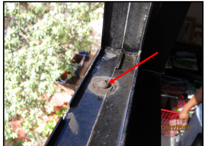
46. DETERIORATED SEALANT AROUND FASTENER IN WINDOW FRAME
