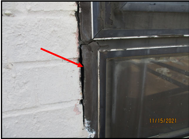
25. DISBONDED AND DETERIORATED SEALANT AT WINDOW PERIMETER
