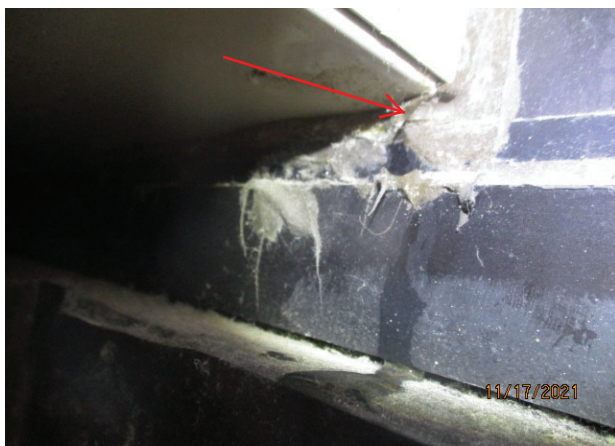
59. SPECIMEN 2.02: WATER INFILTRATION BETWEEN WINDOW FRAME AND PTAC UNIT
