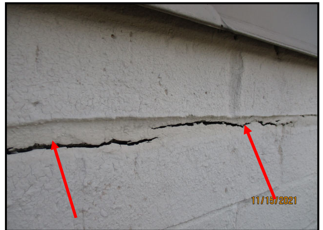
30. DETERIORATED SEALANT IN HORIZONTAL JOINT BETWEEN ADJACENT BRICK UNITS
