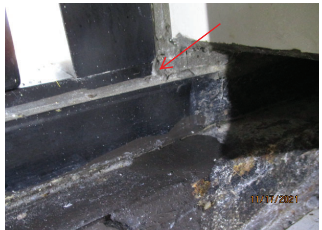
64. SPECIMEN 2.03: WATER INFILTRATION BETWEEN WINDOW FRAME AND PTAC UNIT
