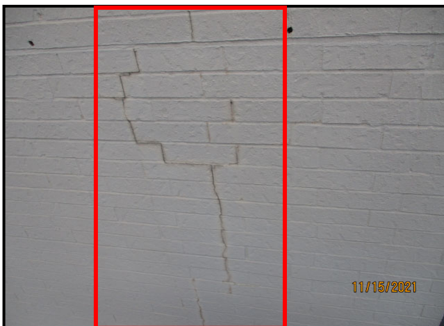
35. STEP CRACK IN BRICK
