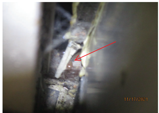
60. SPECIMEN 2.02: WATER INFILTRATION BETWEEN WINDOW FRAME AND PTAC UNIT
