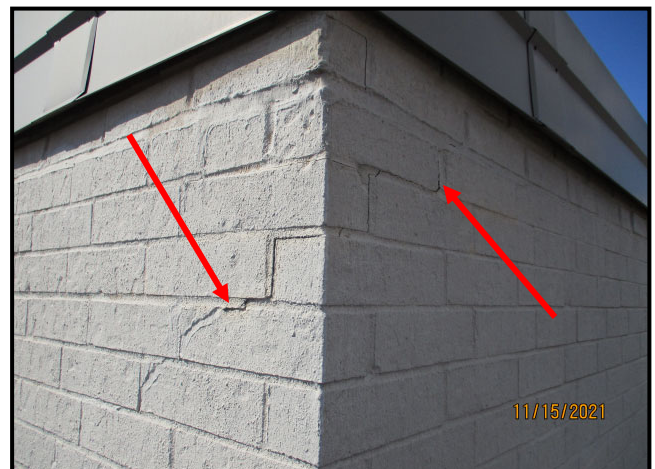
36. STEP CRACK IN BRICK
