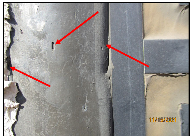
24. DISBONDED AND DETERIORATED SEALANT AT WINDOW PERIMETER
