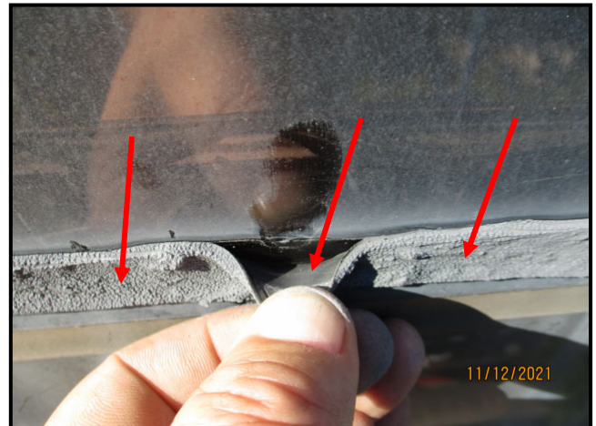
16. DISBONDED/DETERIORATED SEALANT AT EDGE OF WINDOW GLAZING
