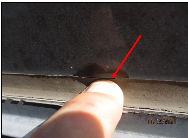
11. DISBONDED SEALANT AT EDGE OF WINDOW INSULATED GLASS UNIT
