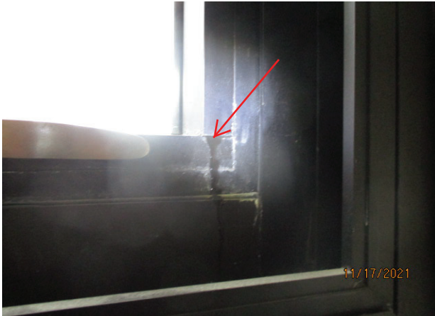
61. SPECIMEN 2.02: WATER INFILTRATION AT BOTTOM CORNER OF OPERABLE WINDOW SASH
