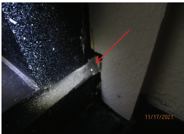
57. SPECIMEN 2.01: WATER INFILTRATION OUTSIDE FRAME OF VERTICAL MULLION
