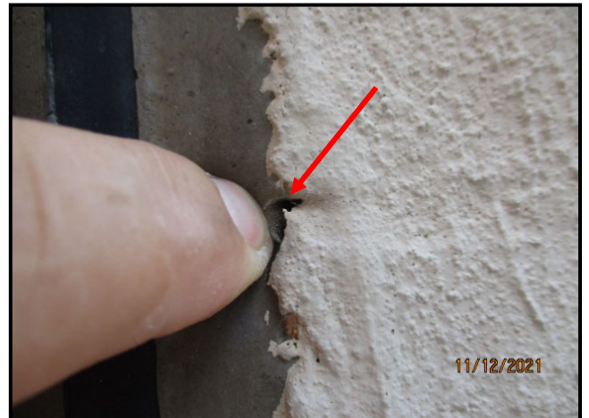
22. DISBONDED SEALANT AT WINDOW PERIMETER
