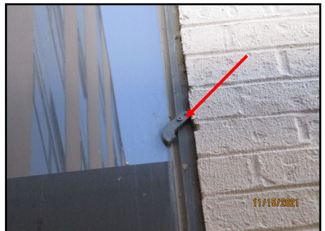
42. GLASS APPARENTLY RETAINED WITH SECTION OF PLASTIC SHIM
