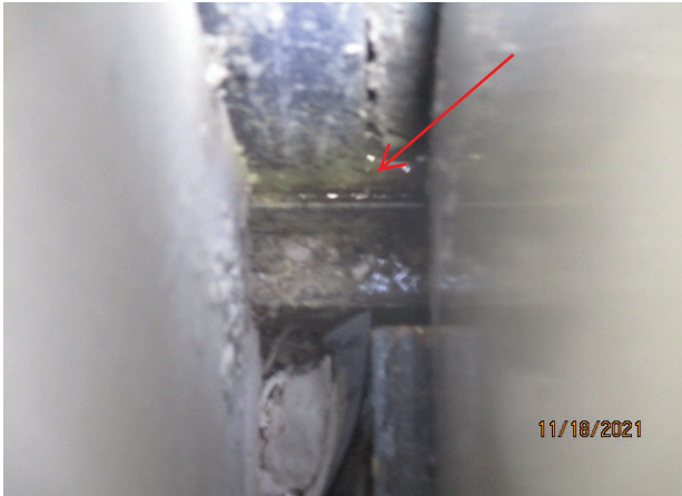
73. SPECIMEN 3.03: WATER INFILTRATION BETWEEN WINDOW FRAME AND PTAC UNIT
