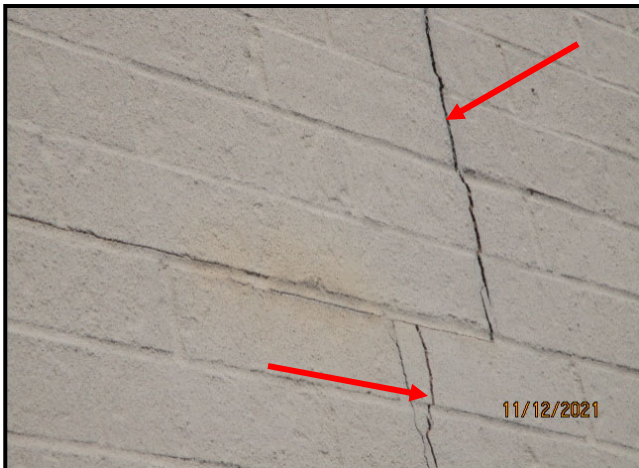
39. VERTICAL CRACKS IN BRICK
