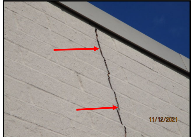
38. VERTICAL CRACK IN BRICK
