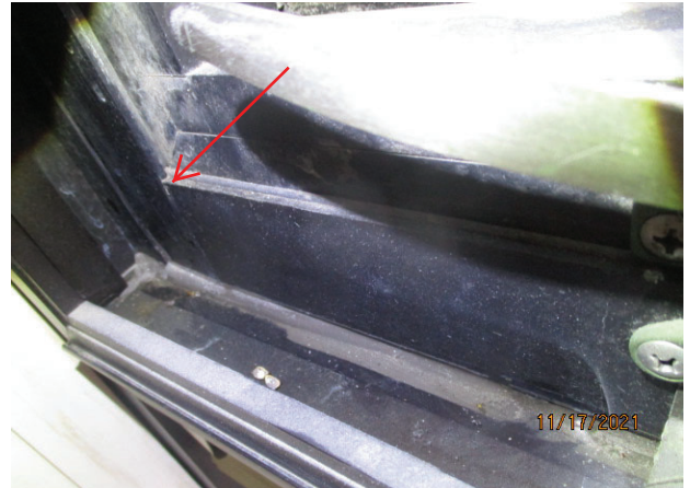
62. SPECIMEN 2.02: WATER INFILTRATION AT BOTTOM CORNER OF OPERABLE WINDOW SASH
