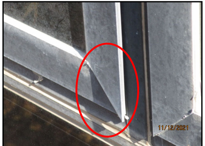
10. MISALIGNED CORNER AT WINDOW SASH
