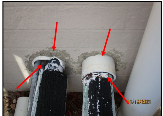
34. DETERIORATED SEALANT BETWEEN WALL PENETRATION AND BRICK UNITS; NO SEALANT BETWEEN PIPES AND PVC SLEEVE
