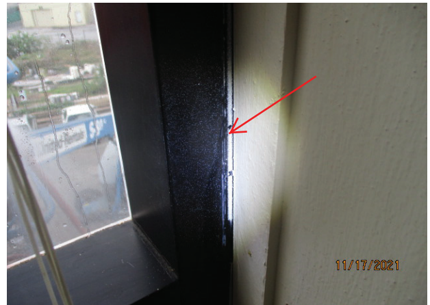
56. SPECIMEN 2.01: WATER INFILTRATION RIGHT SIDE OF WINDOW
