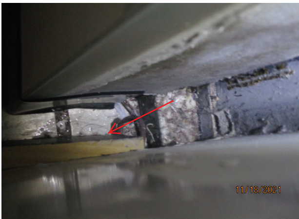
69. SPECIMEN 3.01: WATER INFILTRATION AT LEFT VERTICAL MULLION
