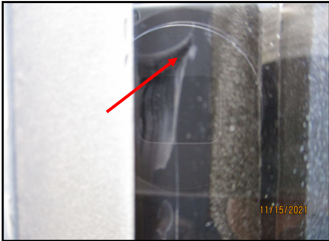
27. VOID IN BED OF STRUCTURAL SEALANT BEHIND WINDOW INSULATED GLASS UNIT
