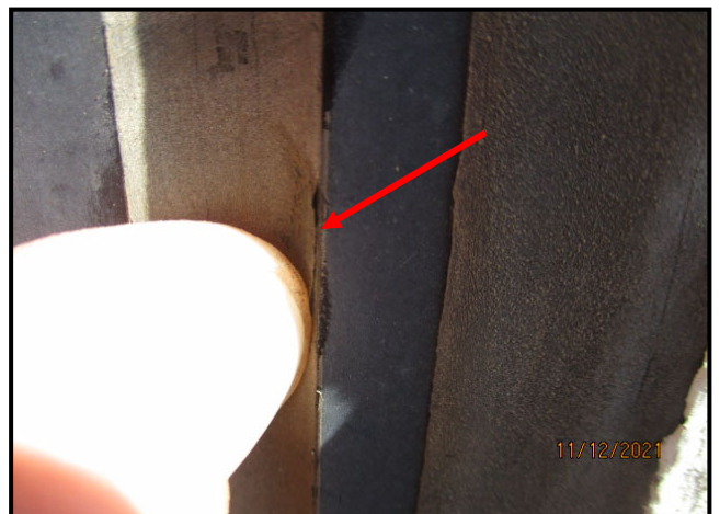
12. DISBONDED SEALANT AT MULLER WINDOW FRAME
