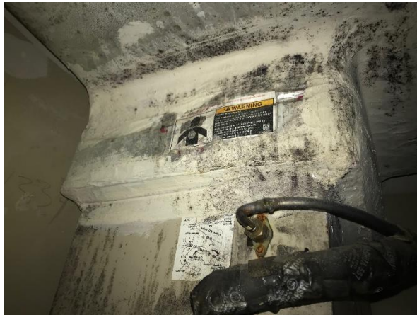
4. White duct insulation seam mastic
