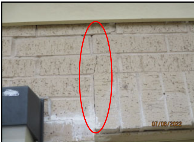
35. TYPICAL CRACK IN BRICK VENEER AT TOP CORNER OF WALL OPENING AT GARAGE; PREVIOUS TUCKPOINTING ADJACENT TO CRACK
