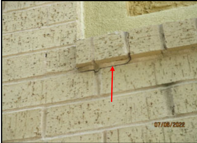
43. CRACK IN MORTAR BETWEEN ADJACENT BRICK UNITS
