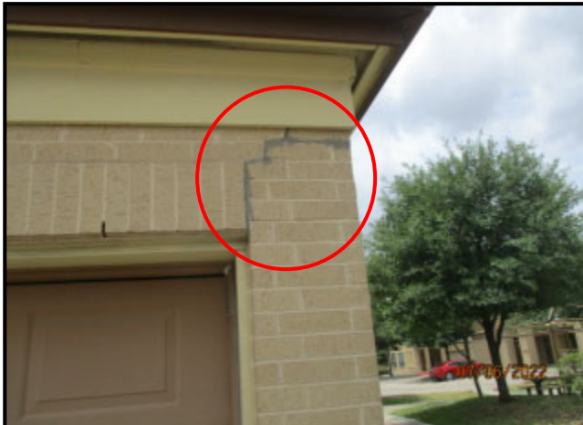
39. TYPICAL STEP CRACK IN BRICK VENEER AT TOP CORNER OF WALL OPENING AT GARAGE
