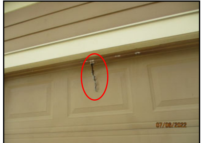
52. DAMAGED GARAGE DOOR PANEL
