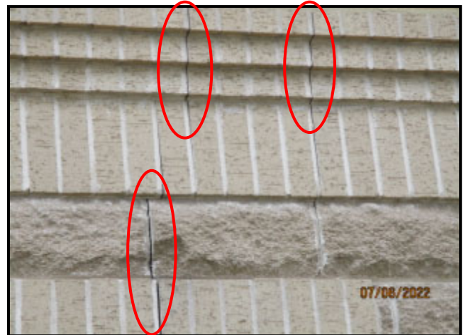
44. CRACKS IN MORTAR BETWEEN ADJACENT BRICK UNITS AND BETWEEN ADJACENT CMU BLOCKS
