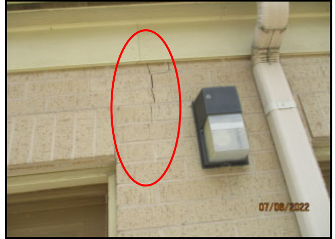
38. TYPICAL CRACK IN BRICK VENEER AT TOP CORNER OF WALL OPENING AT GARAGE
