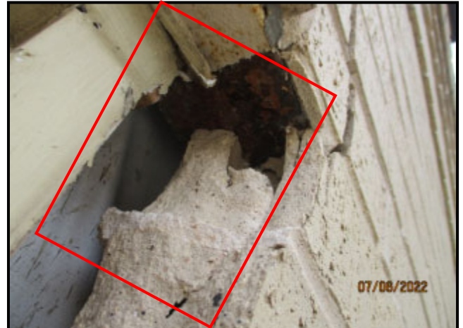
46. SPALLED/DISPLACED BRICK VENEER AT END OF STEEL LINTEL
