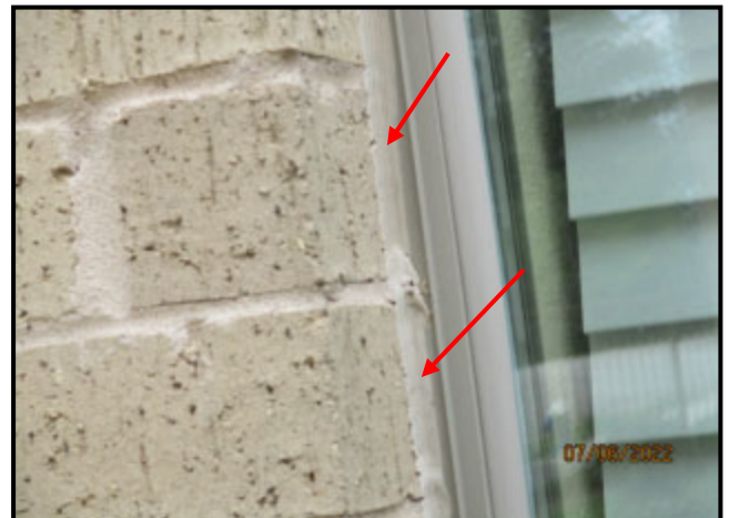
48. DETERIORATED SEALANT AT WINDOW PERIMETER
