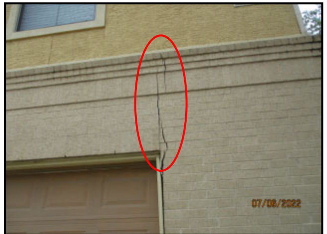
36. TYPICAL CRACK IN BRICK VENEER AT TOP CORNER OF WALL OPENING AT GARAGE
