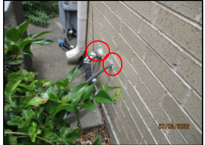
50. DETERIORATED AND MISSING SEALANT AROUND WALL PENETRATIONS
