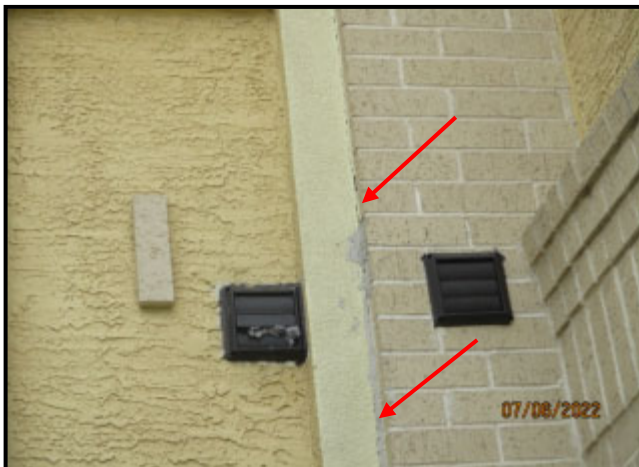
47. DETERIORATED SEALANT AT CONTROL JOINT
