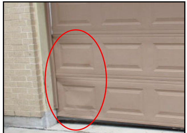
54. DAMAGED GARAGE DOOR PANEL
