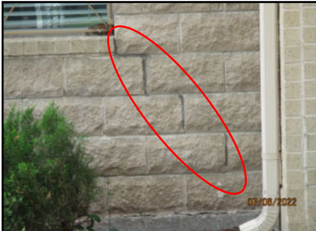
45. TYPICAL STEP CRACK IN CMU VENEER AT BOTTOM CORNER OF WALL OPENING AT AMENTITY CENTER
