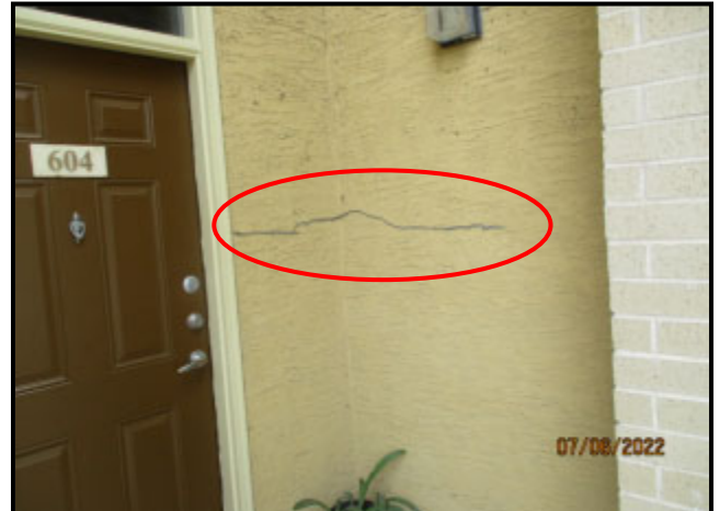
40. TYPICAL CRACK IN STUCCO (sealant had been applied over crack)
