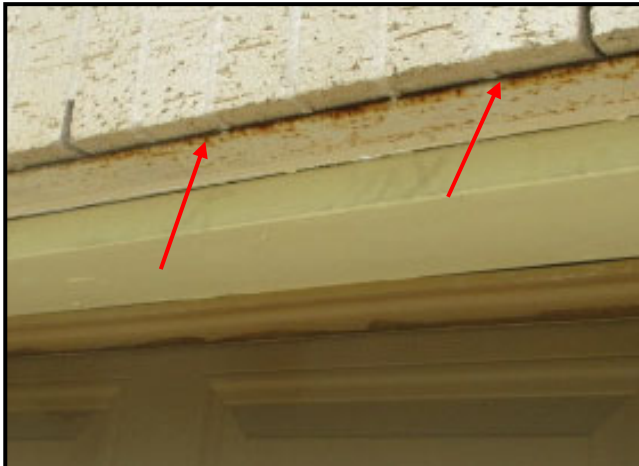
51. CORRODED STEEL LINTEL ABOVE GARAGE WALL OPENING
