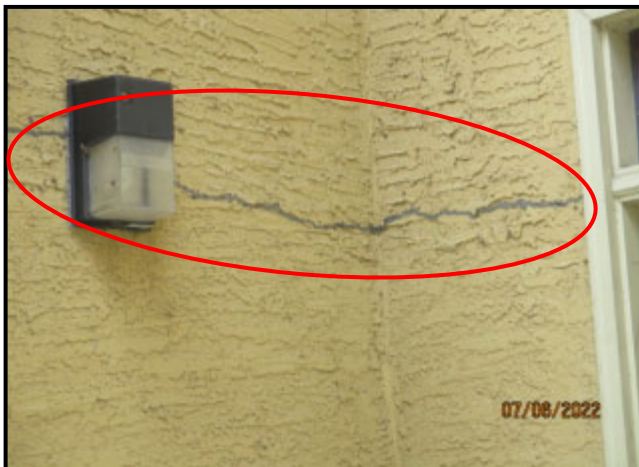
41. TYPICAL CRACK IN STUCCO (sealant had been applied over crack)
