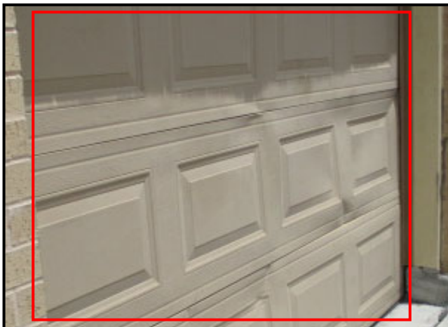
53. DAMAGED GARAGE DOOR PANELS
