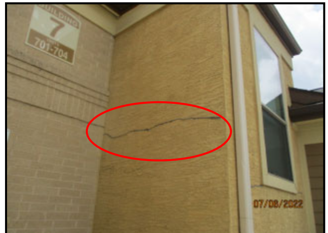
42. TYPICAL CRACK IN STUCCO (sealant had been applied over crack)
