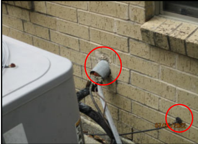
49. DETERIORATED AND MISSING SEALANT AROUND WALL PENETRATIONS
