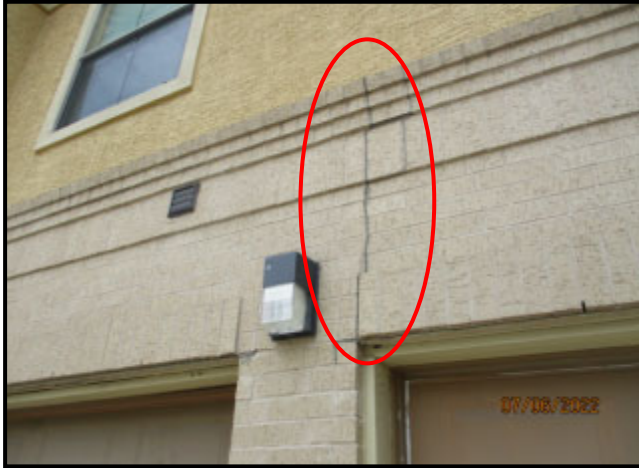
37. TYPICAL CRACK IN BRICK VENEER AT TOP CORNER OF WALL OPENING AT GARAGE
