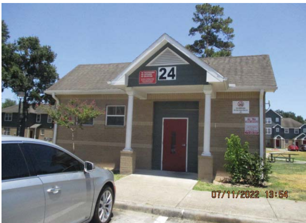
11. BUILDING NO. 24: OVERVIEW
