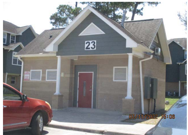
10. BUILDING NO. 23; OVERVIEW
