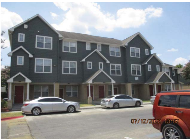
5. BUILDING TYPE 3, BUILDING NO. 3; OVERVIEW - BUILDING NOS. 10 AND 18 ARE SIMILAR
