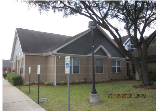
2. BUILDING NO. 2: OVERVIEW
