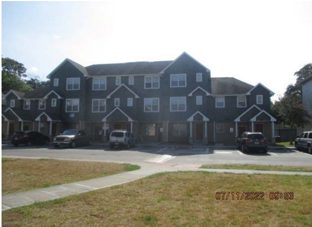
7. BUILDING TYPE 5, BUILDING NO. 21; OVERVIEW
