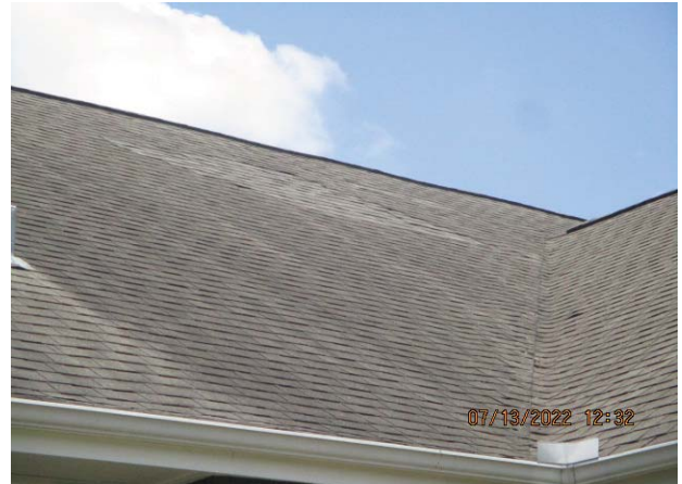
14. BUILDING NO. 2: TYPICAL SHINGLE REPAIR
