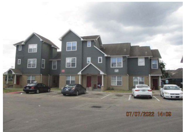
4. BUILDING TYPE 2, BUILDING NO. 13; OVERVIEW
