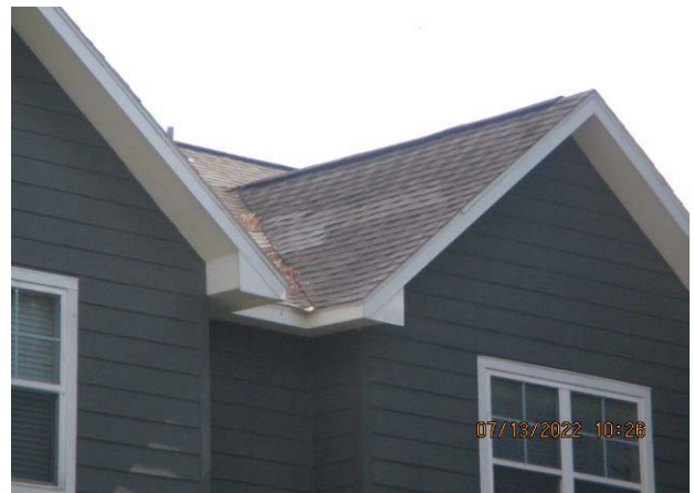
12. BUILDING NO. 6: TYPICAL SHINGLE REPAIR
