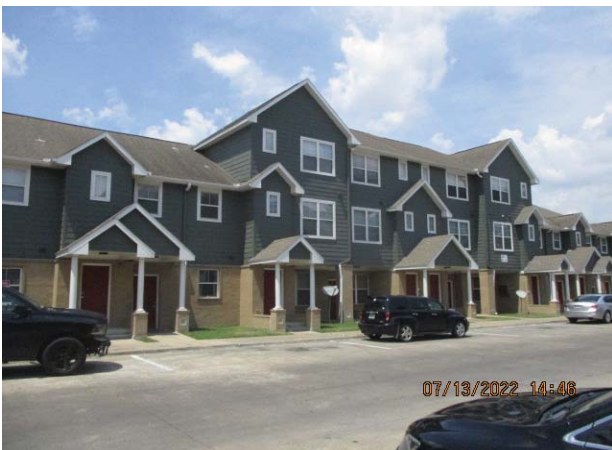
3. BUILDING TYPE 1, BUILDING NO. 7, OVERVIEW; BUILDING NOS. 8, 12, 15, 16, AND 19 ARE SIMILAR
