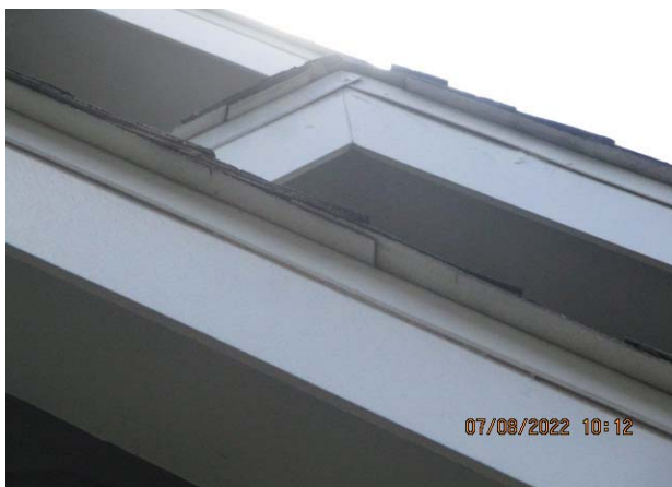
29. BUILDING NO. 15: SHINGLE INSERTED ALONG RAKE EDGE INSTALLED WITH BACKWATER LAP
