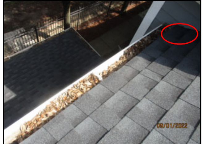
110. KICK-OUT FLASHING NOT INSTALLED AT EDGE OF ROOF ALONG RISE WALL
