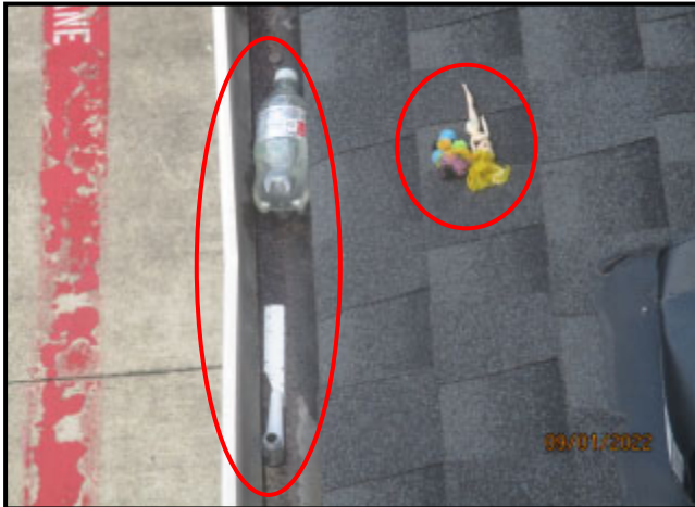
97. DEBRIS IN GUTTER AND ON ROOF SURFACE
