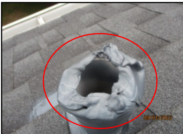
95. LEAD FLASHING NOT PROPERLY FOLDED INSIDE OF PLUMBING VENT PIPE
