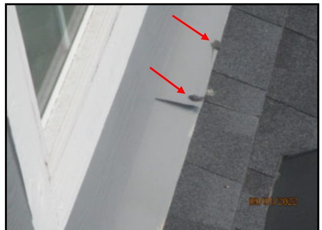
102. NAILS BACKING OUT OF SHEET METAL HEAD WALL FLASHING
