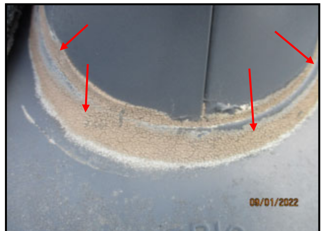
108. DETERIORATED SEALANT AT SHEET METAL JOINT
