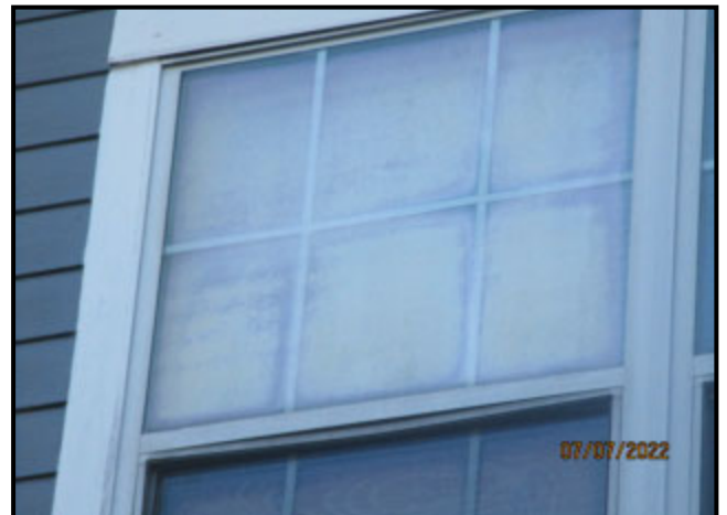
42. TYPICAL MOISTURE/STAINS BETWEEN LITES OF GLASS
