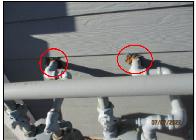
52. DETERIORATED SEALANT AT WALL PENETRATIONS (TYPICAL THROUGHOUT)
