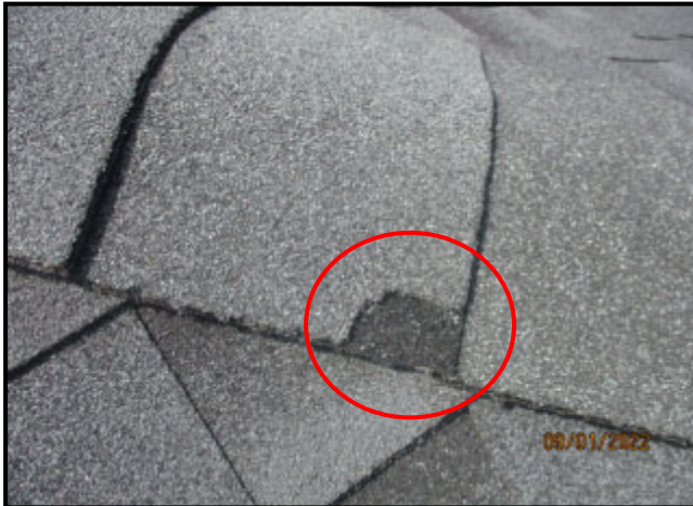
85. DAMAGED SHINGLE
