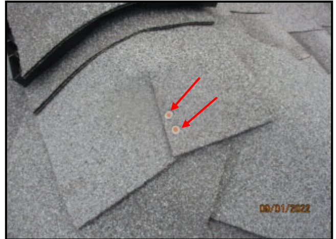
92. EXPOSED AND CORRODED NAILS
