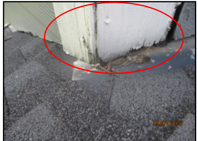
100. DETERIORATED WOOD TRIM
