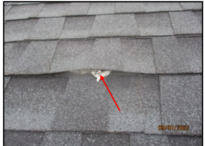
106. DEBRIS BENEATH SHINGLE
