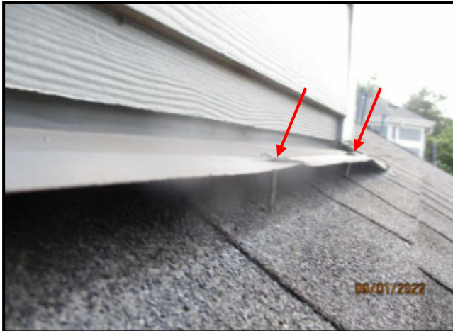
103. NAILS BACKING OUT OF SHEET METAL HEAD WALL FLASHING
