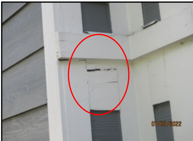
59. DETERIORATED WOOD TRIM
