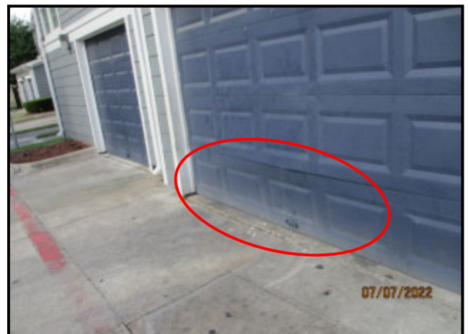
48. DAMAGED GARAGE OVERHEAD DOOR PANELS
