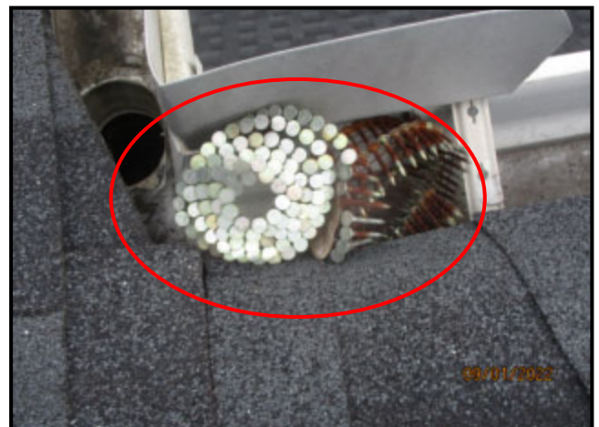
96. DEBRIS IN GUTTER
