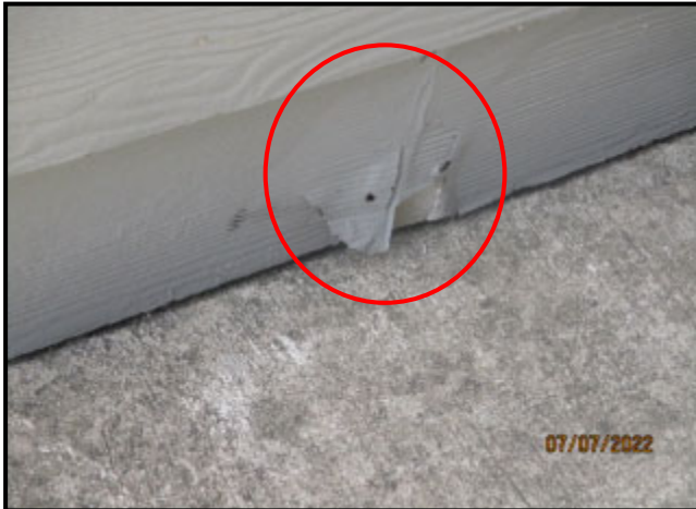
55. DAMAGED FIBER-CEMENT SIDING
