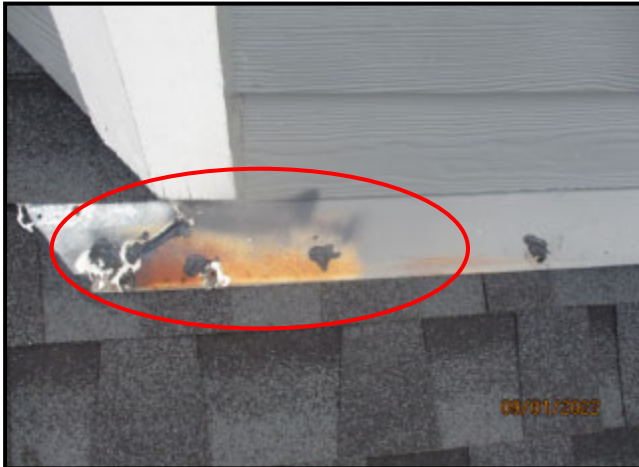
91. CORRODED SHEET METAL HEAD WALL FLASHING
