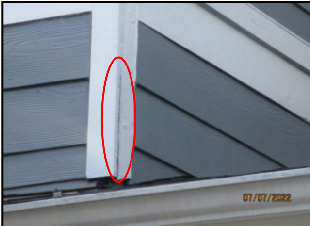
57. DETERIORATED WOOD TRIM
