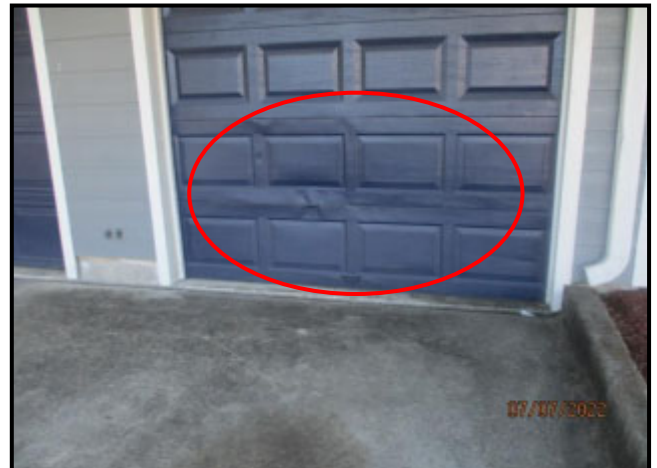
46. DAMAGED GARAGE OVERHEAD DOOR PANELS
