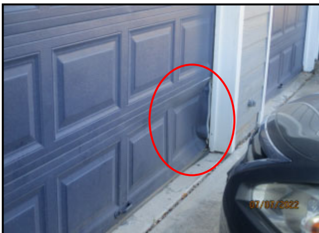
47. DAMAGED GARAGE OVERHEAD DOOR PANEL
