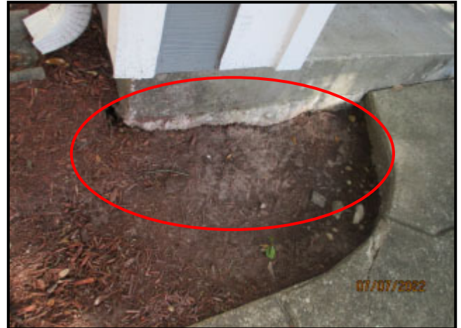
62. BUILDING 4/5: SOIL UNDERMINED AT FRONT ENTRY PATIO
