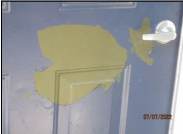
49. BUILDING NO.24: PAINT NOT ADEQUATELY BONDED (PEELING FROM UNDERLYING COATING)
