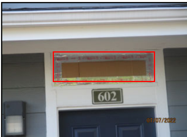
53. BUILDING NO.6: MISSING/BROKEN GLASS IN WINDOW ABOVE DOOR
