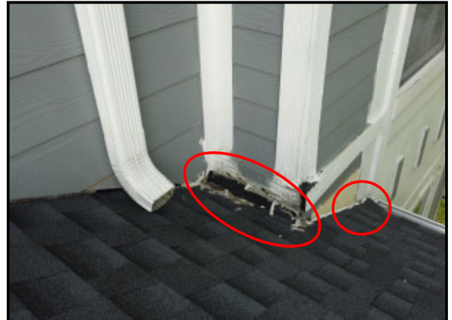
112. KICK-OUT FLASHING NOT INSTALLED AT EDGE OF ROOF ALONG RISE WALL
