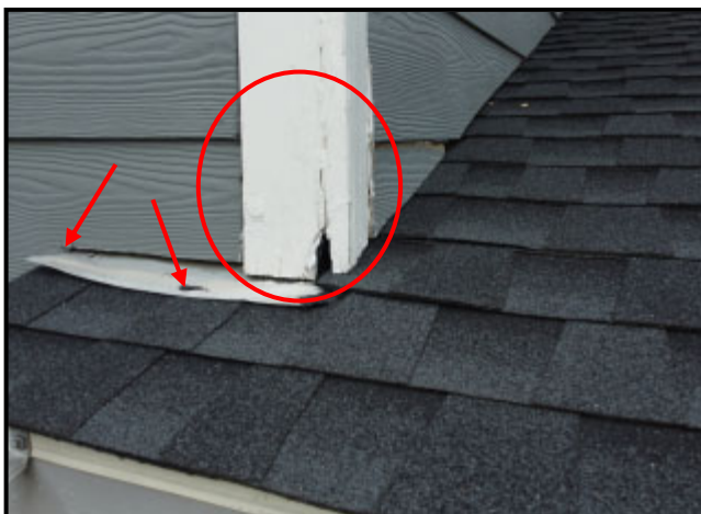
101. NAILS BACKING OUT OF SHEET METAL HEAD WALL FLASHING; DETERIORATED WOOD TRIM
