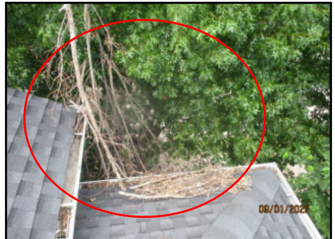
88. TREE LIMBS ON ROOF AND IN GUTTER
