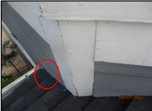
111. KICK-OUT FLASHING NOT INSTALLED AT EDGE OF ROOF ALONG RISE WALL
