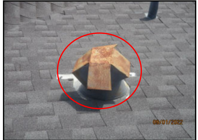
98. CORRODED SHEET METAL VENT
