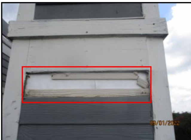
89. DAMAGED/MISSING SIDING
