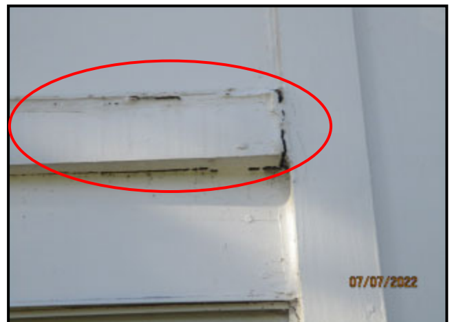
54. DAMAGED FIBER-CEMENT SIDING
