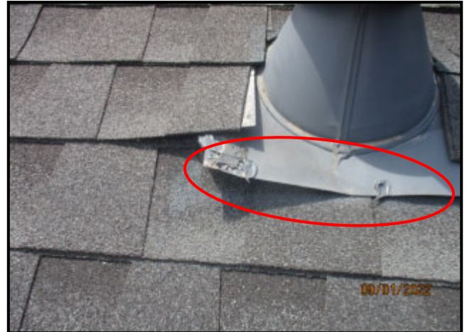
104. FLANGE OF VENT NOT SECURED
