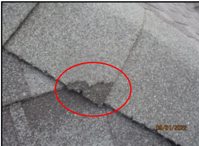
87. DAMAGED SHINGLE
