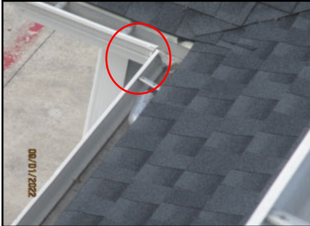
109. SHEET METAL DEFLECTOR NOT INSTALLED TO GUTTER AT BOTTOM OF VALLEY
