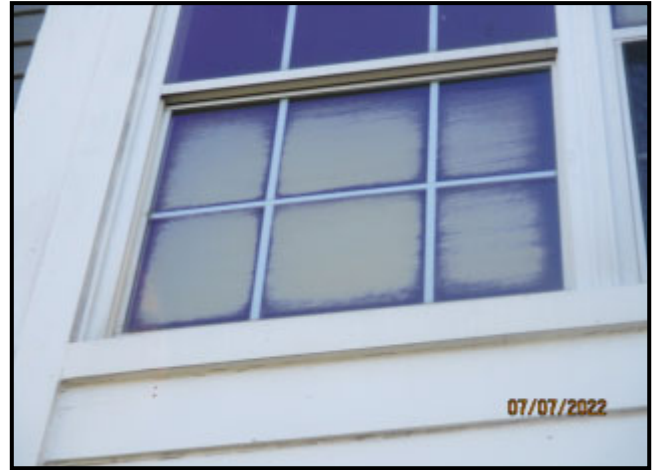
44. TYPICAL MOISTURE/STAINS BETWEEN LITES OF GLASS
