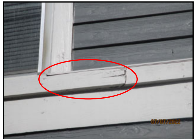
60. DETERIORATED WOOD TRIM
