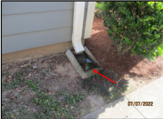
61. CONCRETE SPASH BLOCK IMPROPERLY ORIENTED
