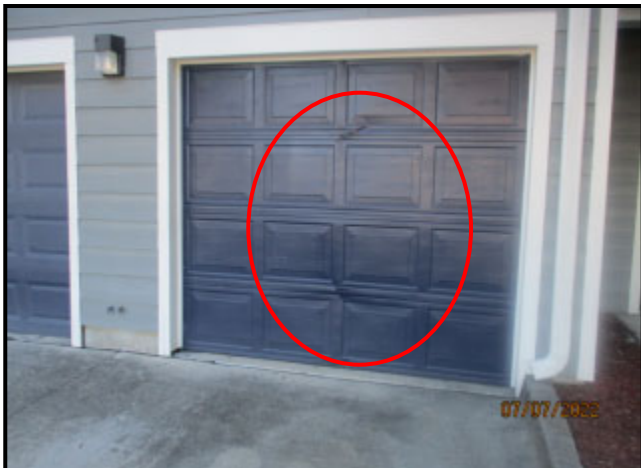
45. DAMAGED GARAGE OVERHEAD DOOR PANELS
