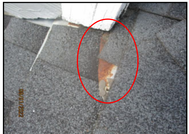
90. CORRODED SHEET METAL STEP FLASHING
