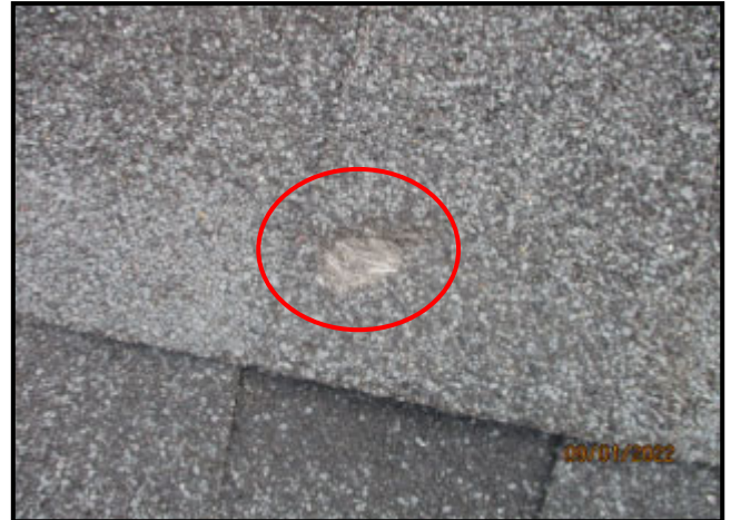
86. DAMAGED SHINGLE
