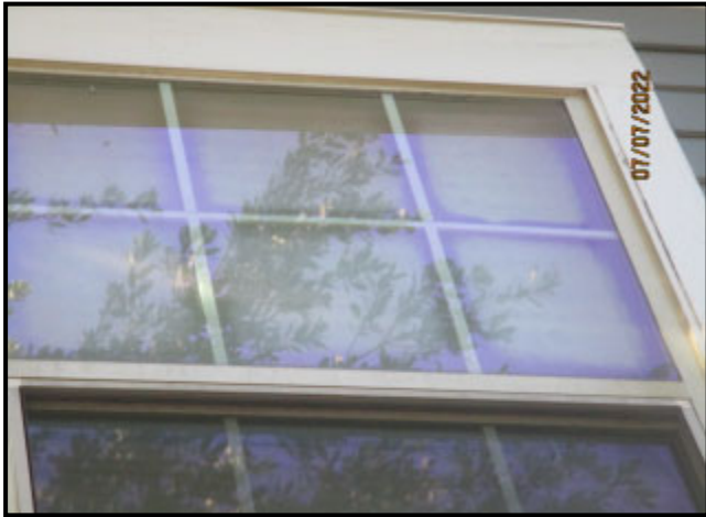
43. TYPICAL MOISTURE/STAINS BETWEEN LITES OF GLASS
