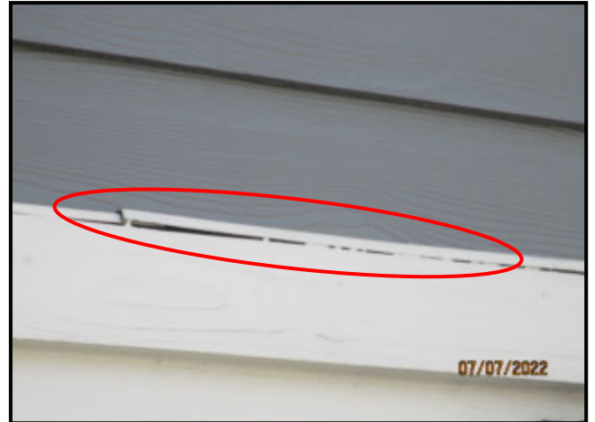
56. LOOSE SHEET METAL THROUGH WALL FLASHING
