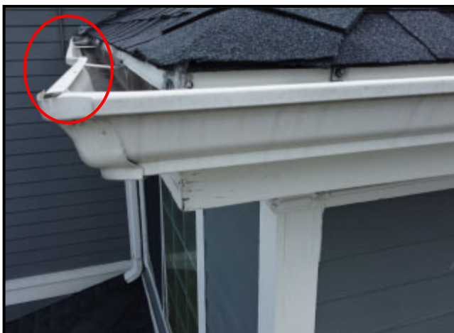
107. DAMAGED GUTTER
