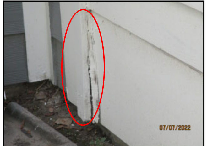
58. DETERIORATED WOOD TRIM
