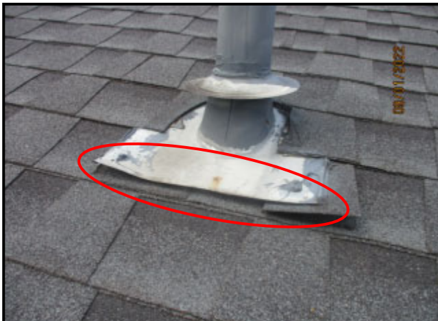
105. FLANGE OF VENT NOT SECURED
