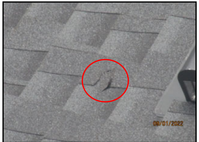
84. DAMAGED SHINGLE
