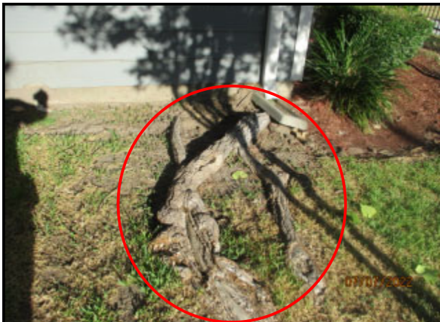
63. BUILDING NO.6; ROOT UNDERMINING FOUNDATION
