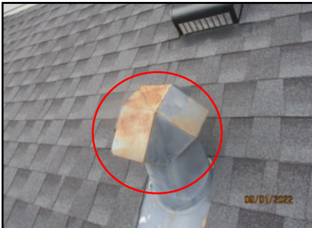
99. CORRODED SHEET METAL VENT
