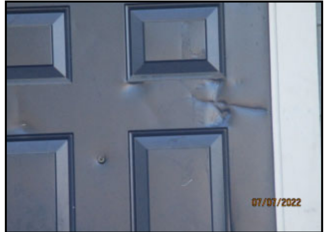
50. BUILDING NO.4/5: DAMAGED ENTRY DOOR
