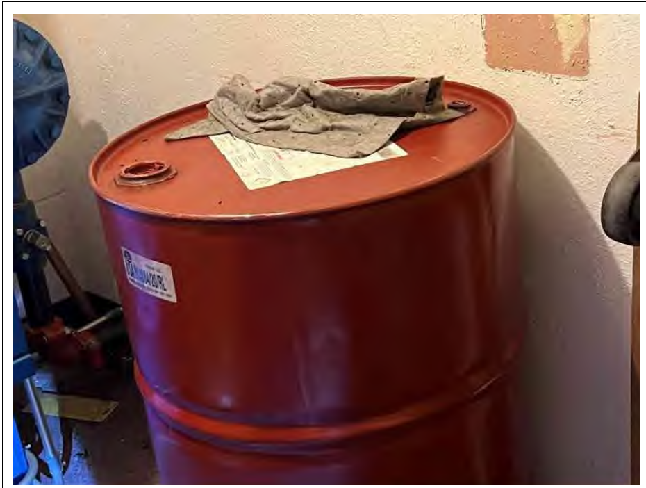
PHOTO #20 DESCRIPTION: Chemical stored in the mechanical room
