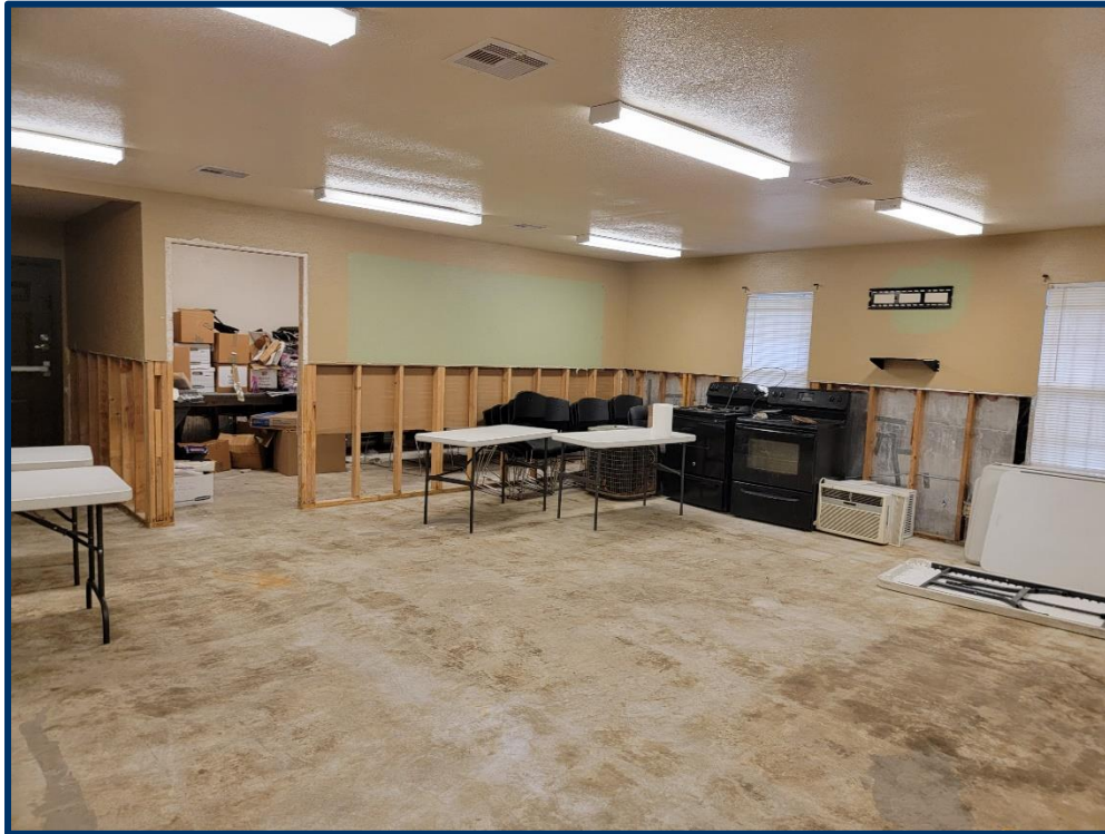
Interior view of the clubhouse/management office
