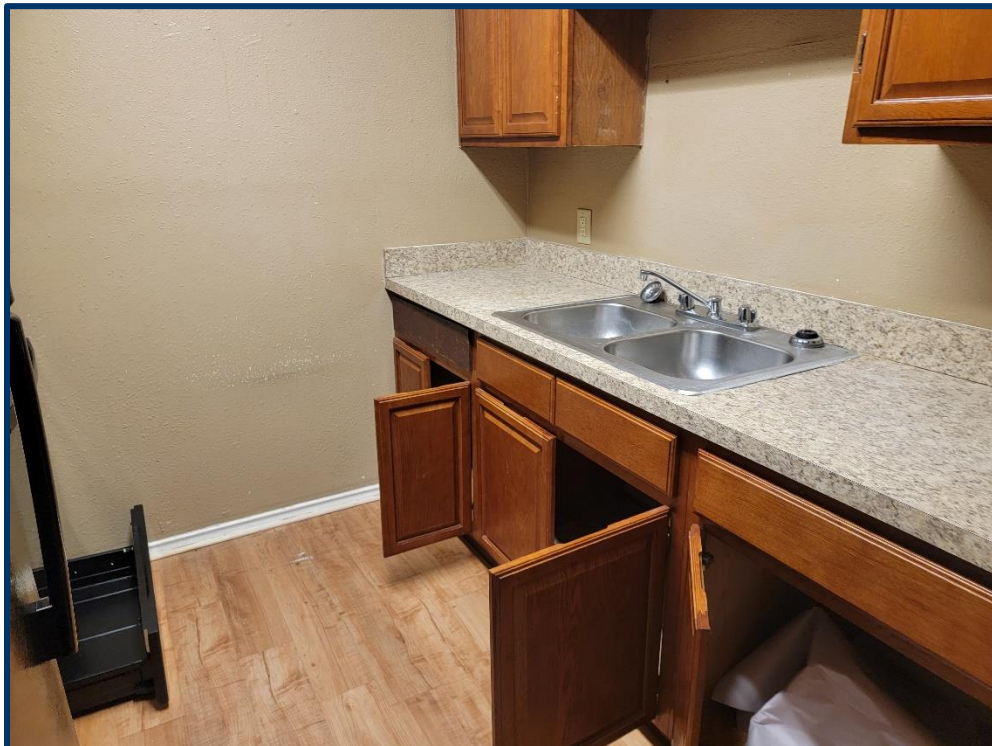
View of one of the recently vacated units – Kitchen area
