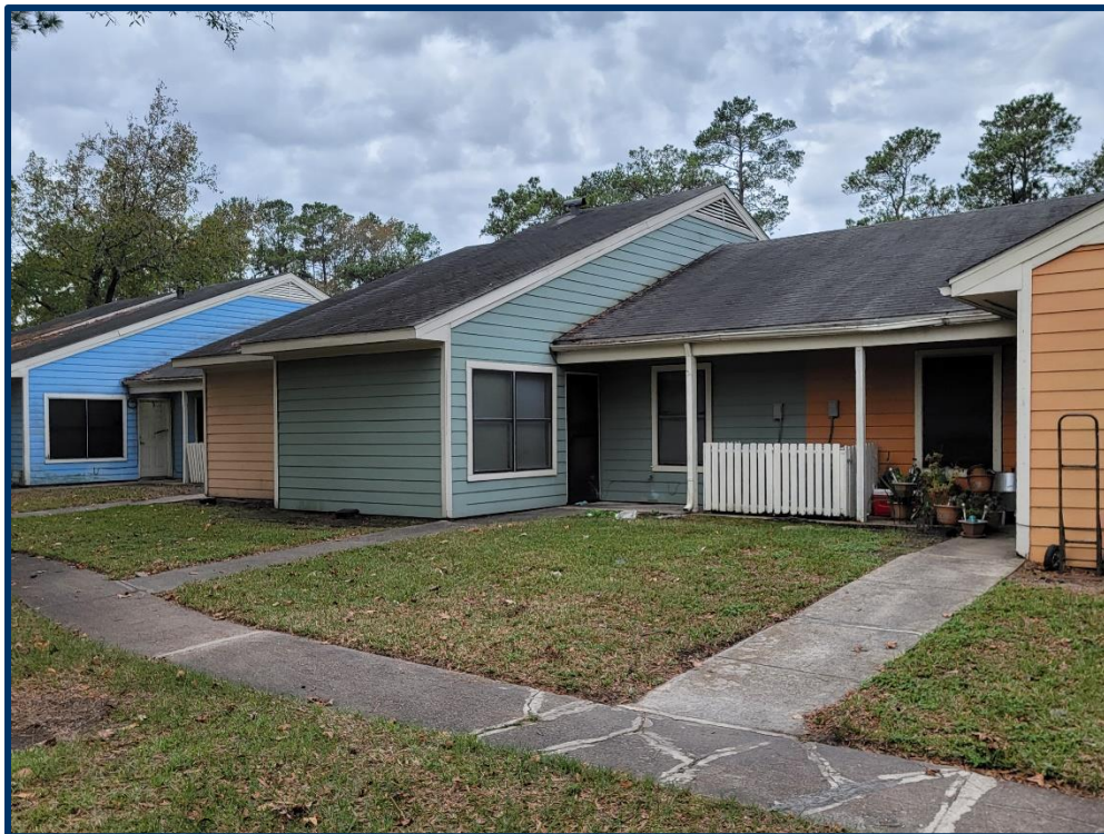
Typical exterior view of the residential units
